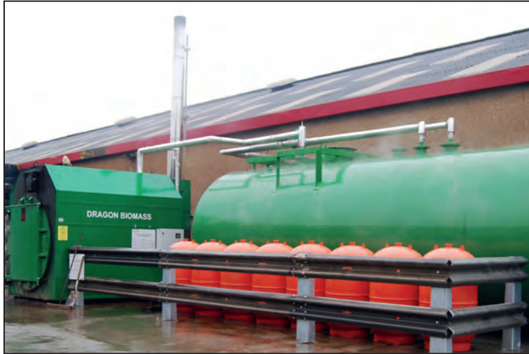
Above: Heating the new paint facility
