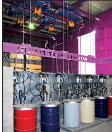
Above: Paint pump station & overhead monorail
